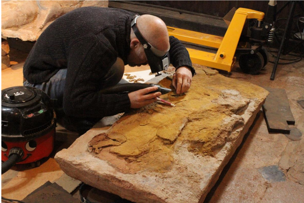
Plate 34: repairs to stone in progress
