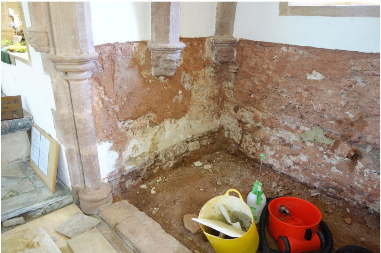
Plate 11 The lower walls of the niche, plaster removed
