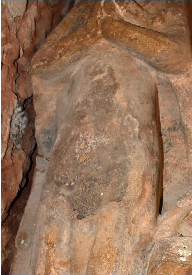
Plate 25 left: large grey cement repair on the lady's gown
