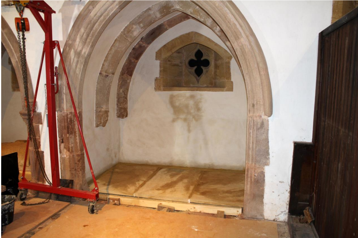
Plate 38: New Ham Hill stone floor laid and recess re-plastered and limewashed
