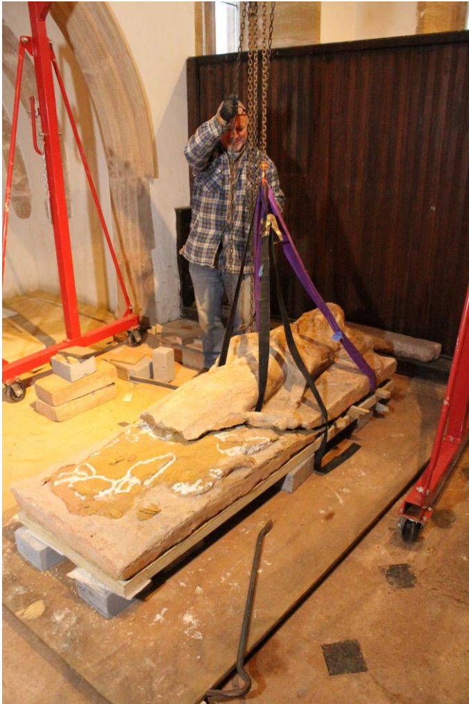
Plate 36: the effigy being reassembled with lifting gear
