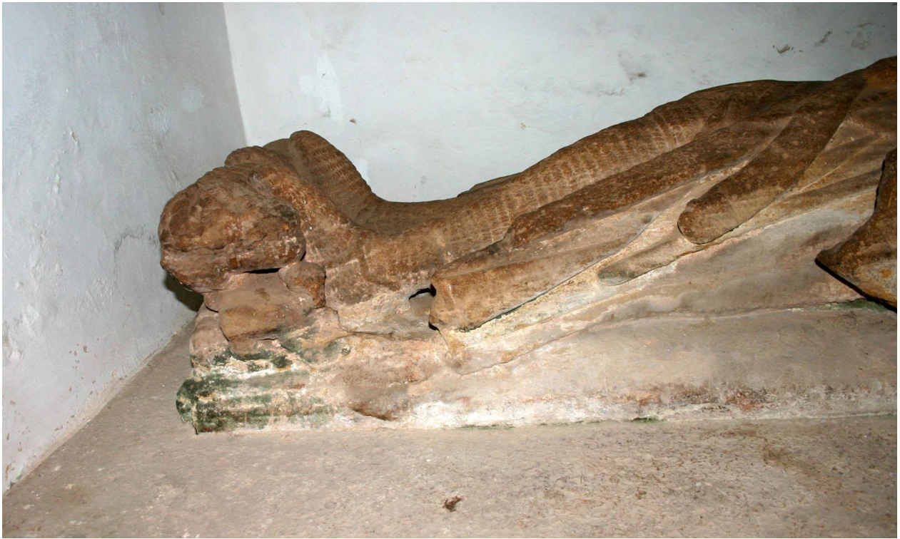
Plate 3 the foot end of the effigy before work, showing damp and growth
